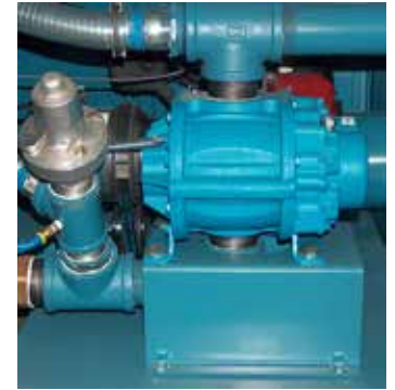
Positive Displacement Blower w/150 CFM @ 5 psi
